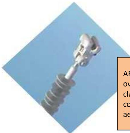
AR Clamps are sized to the conductor and installed over line guards. The articulating feature lets the clamps rotate through large angles, allowing the conductor to twist. This dynamic motion dumps off aerodynamic lift and reduces galloping motion.
