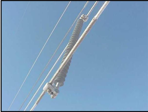
An anti-galloping spacer damper, this solution for transmission lines provides galloping and vibration control in addition to maintaining separation between phase conductors when the predicted galloping amplitude exceeds the available clearance. The AR Spacer Twister has two articulating clamps at each end of a polymer insulator. AR Spacer Twister may be used in combination with other AR anti-galloping dampers.
