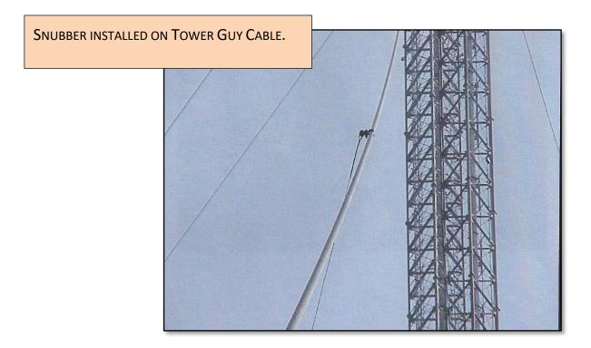
AR<sup>®</sup> Snubber Systems are anti-galloping dampers. Installed horizontally on the guy cable, the Clamp can rotate towards the ground up to 90 degrees. This twisting action helps arrest the galloping motion.
