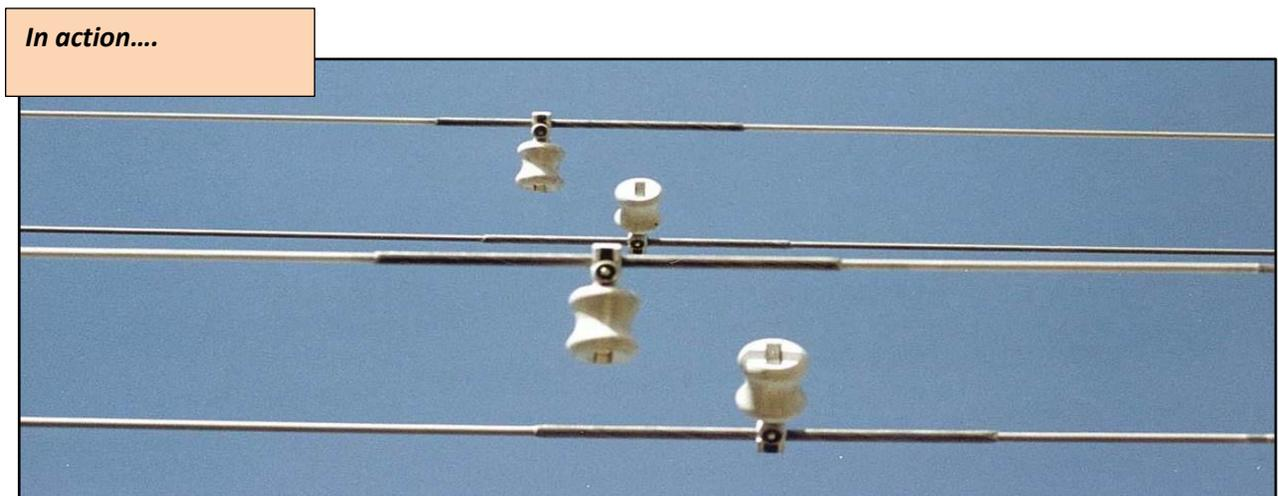
**AR TWISTER | MOD3.** In each span, one damper is clamped first to the Armor Rods then secured to the conductor. The final position depends upon the torsional stiffness of the conductor, previously calculated. The final position of 90 to 120 degrees from vertical is ideal.
