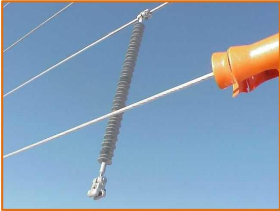
A vibration control and spacer damper, this solution for lighter-weight transmission lines works in concert with AR antigalloping dampers to control galloping AND maintain separation between phase conductors when the predicted galloping amplitude exceeds the available clearance. The AR Spacer Twister has two articulating clamps at each end of a polymer insulator.
